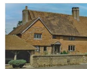
Brick dwarf walls
